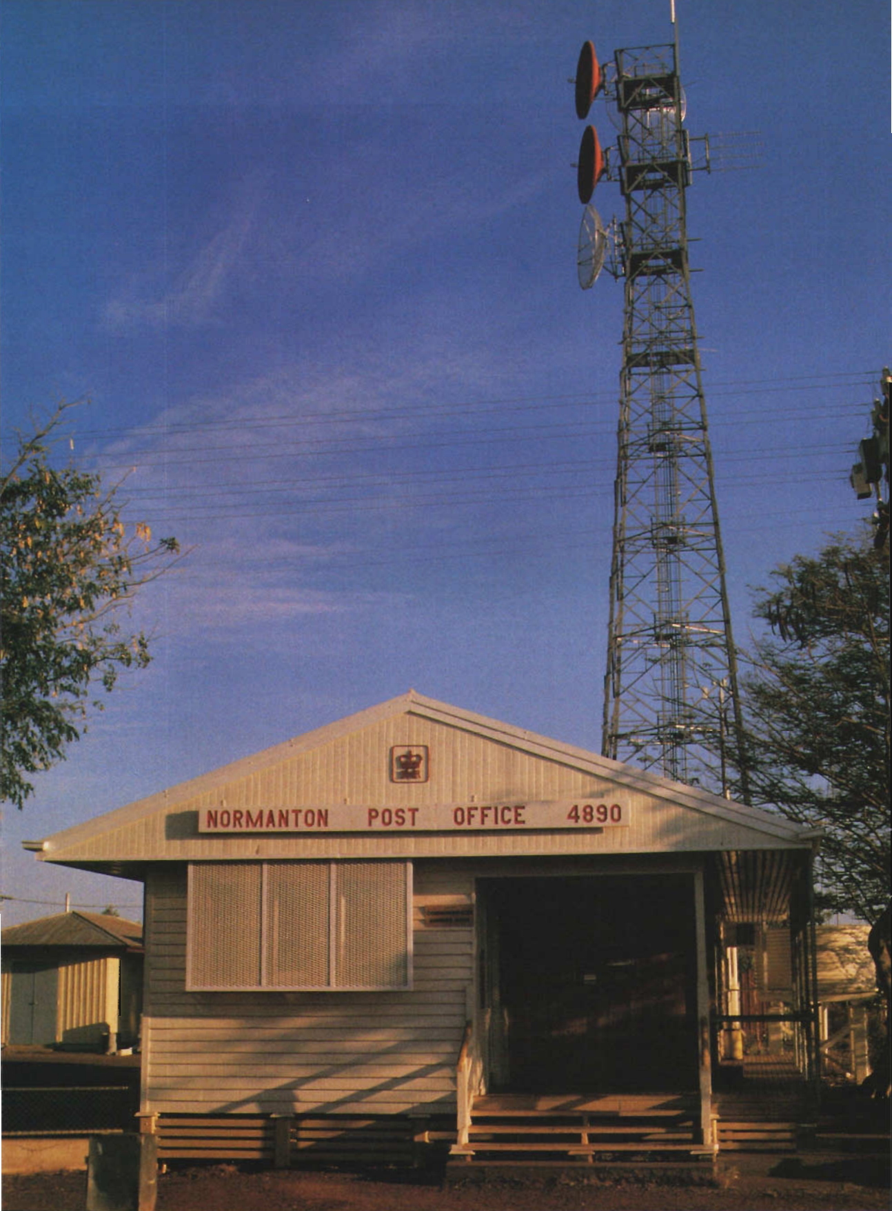
Communications centre in the far north
