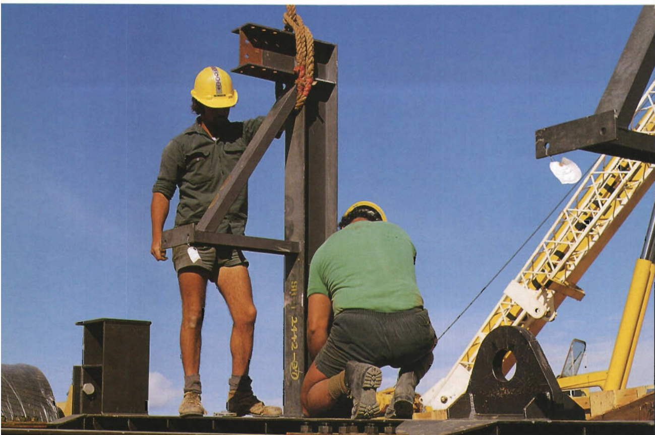
Building workers on a construction site
